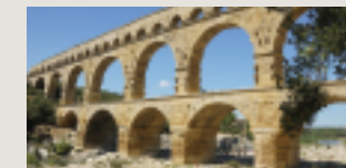
312 B.C. – 226 A.D. Roman Aqueducts, Italy
